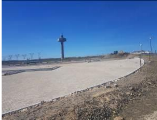
Image 2: Progress of car park extension.
