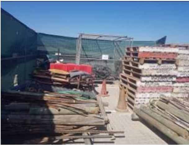
Image 10: Storage of waste within the site camp.
