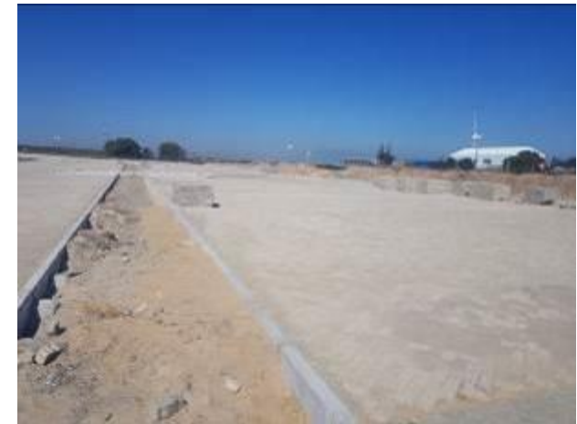
Image 6: Curbing and laid paving.
