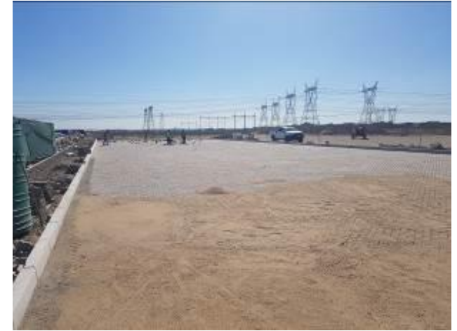
Image 12: Unlaid area, awaiting paving.
