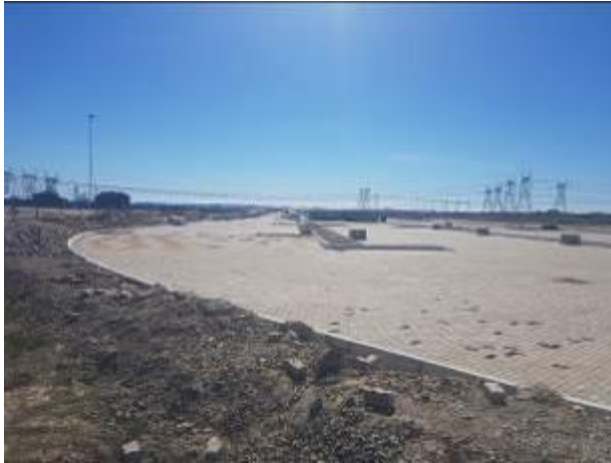
Image 1: Progress of car park extension.
